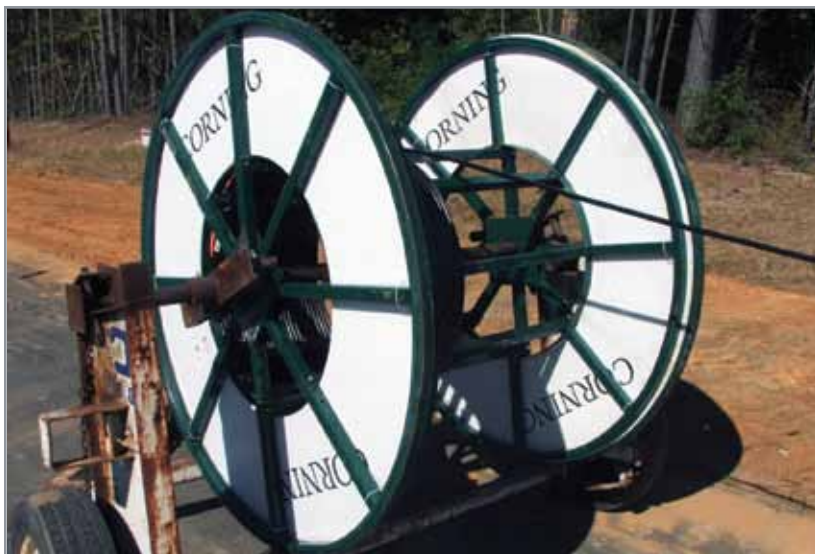
Deploying FlexNAP System via Stationary Reel Method | Photo NS271
