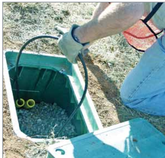
Installation of an OptiSheath Terminal | Photo ACC215
