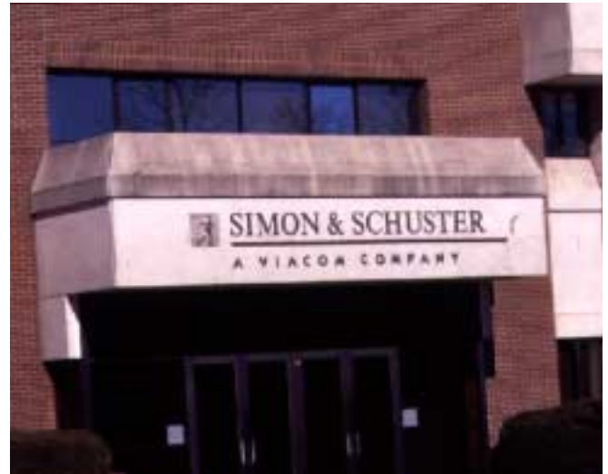
Simon & Schuster's Data Center in Old Tappan, N.J.
