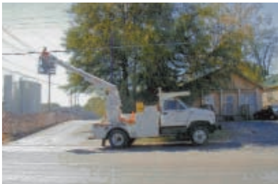
Atlantic Engineering FTTH Installation
